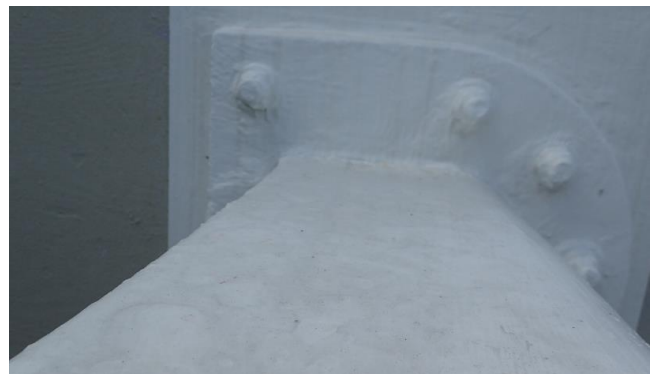
Fig. 2. Flanges after Silicone Protective Coating application
