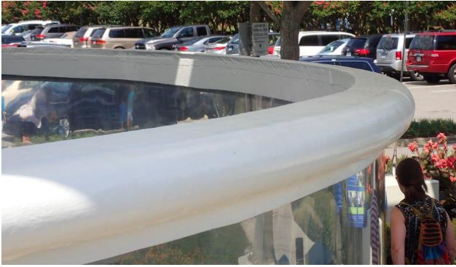
Fig. 3. Seal tank rim after Silicone Protective Coating application
